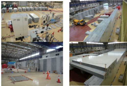
Construction of the radiation shield is on going and will be completed in the end of this September
